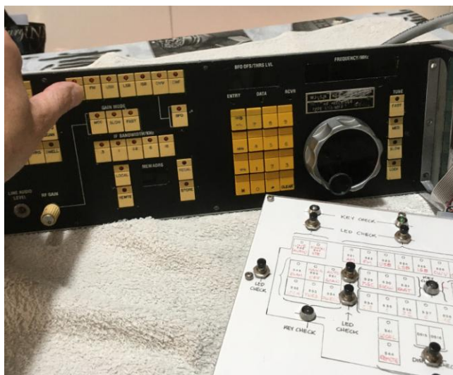
Figure 35: Another switch check that has failed.
