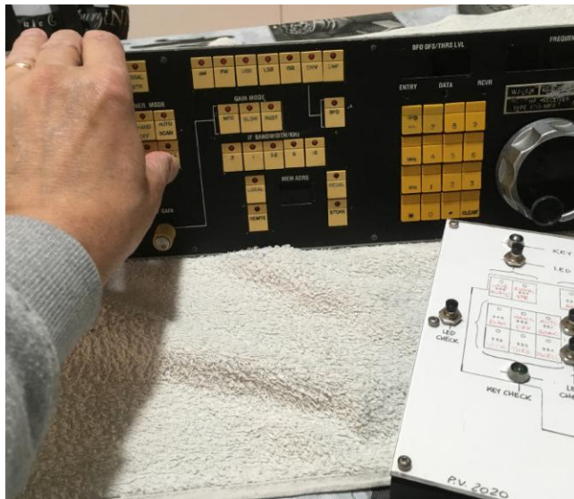
Figure 34: A failed switch check.
